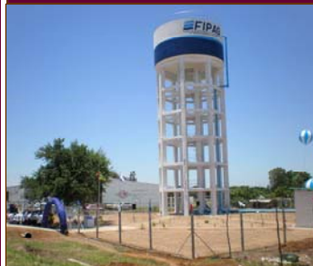
Water Tank for urban water supply in Maputo, Mozambique
