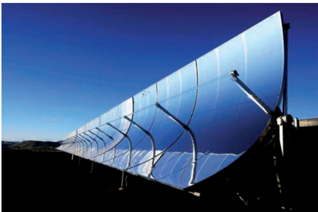
Parabolic trough with mirrors to collect solar energy
