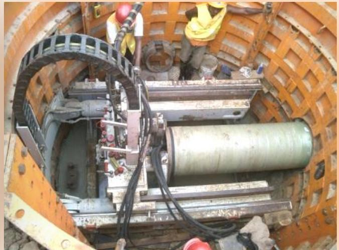
Installation of sewer pipes by micro-tunnelling
