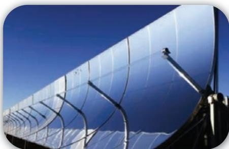
The Xina Solar One Project entails the design, construction, operation and maintenance of a concentrated solar power plant with installed capacity of 100 MW located in the Northern Cape Province. The plant will use parabolic trough technology and a superheated steam cycle with a storage
