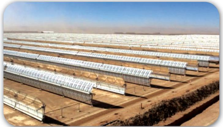
Ouarzazate phase I is already well underway with the first 160 MW solar power plant (NOORo I) expected to be operational by late-2015. The objective of Phase II is to achieve a total capacity of approximately 500 MW by constructing two new
