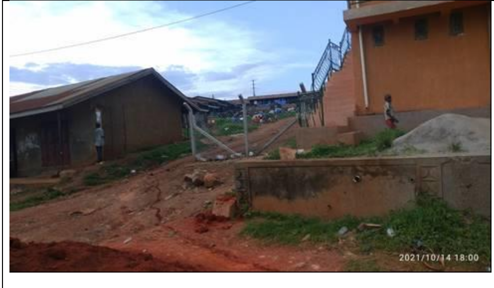
FIGURE 3-1: TOILET FACILITIES IN KIBAALÉ TOWN
