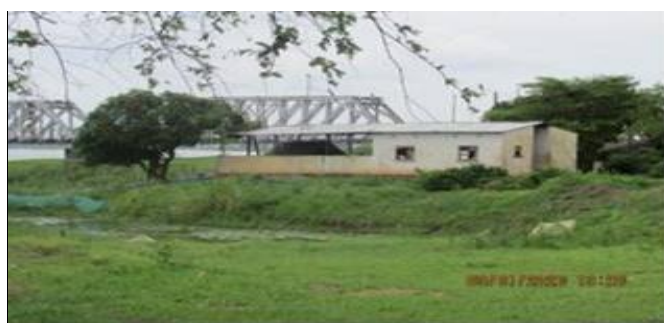
Figure 1: Existing structure on Site
