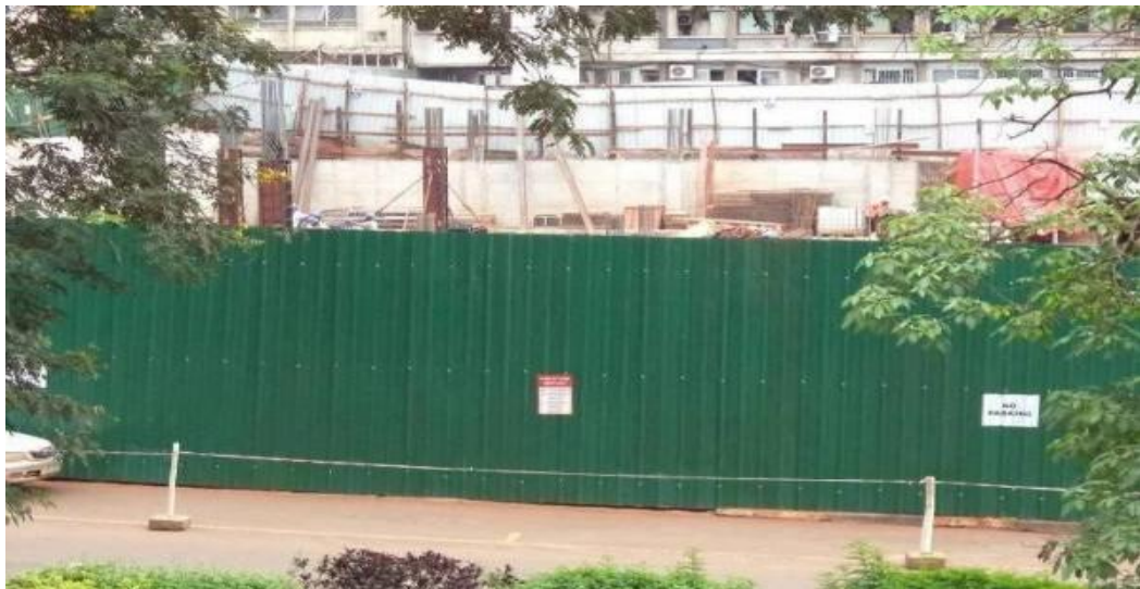
Figure 7: Construction site sealed off with corrugated galvanized iron sheets (CGI).
