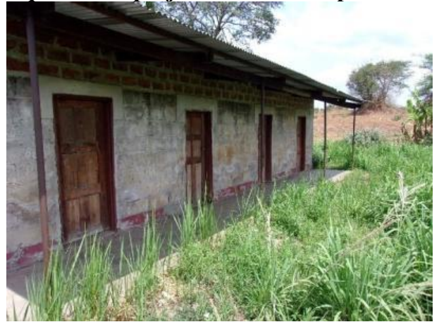
Figure 9: Storage facility structure at Kivuku Aquaculture service centre.
