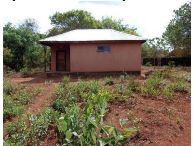
Figure 15: Storage facility structure at Nkenyauna Aquaculture Park project site
