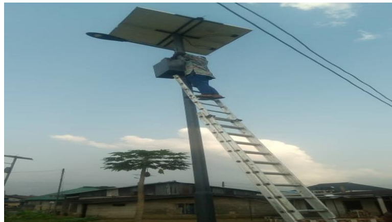
Njuru – Installation of Solar Panel for street lighting
