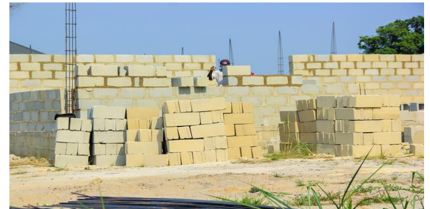
Elenwo – Construction of Division Police HQ
